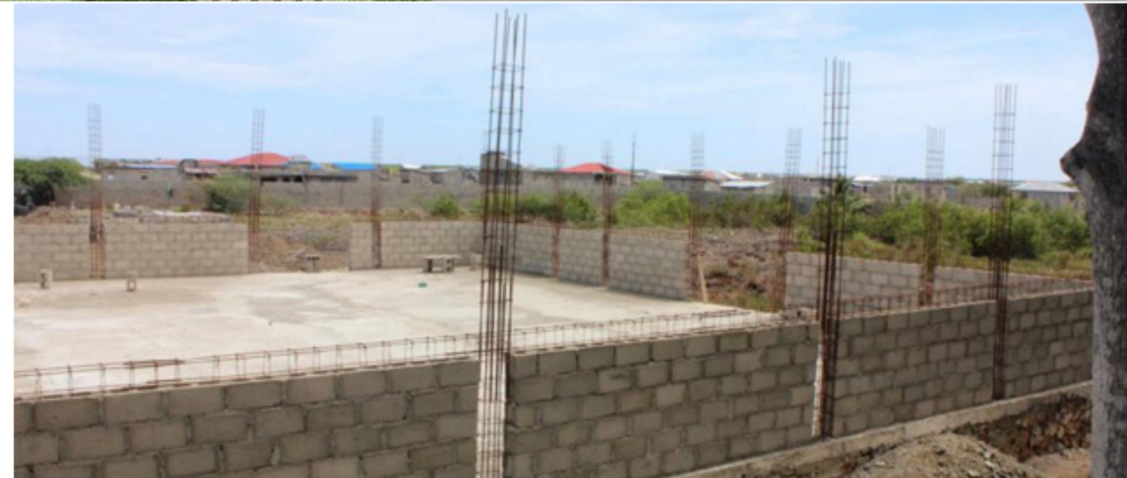
Current progress as of July 2015
